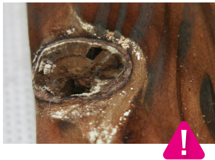
Knot breakouts – up to 20% permitted in intermittent cases
